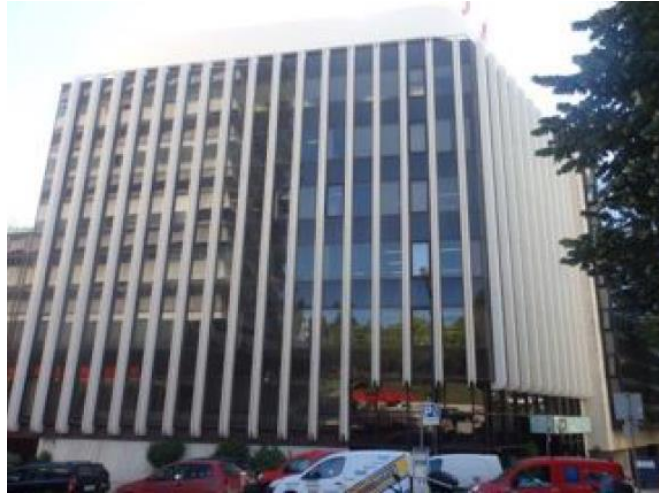
Figure 25: Lisbon Building C's office building
