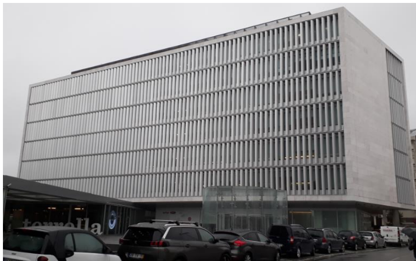
Figure 13: Porto B's office building
