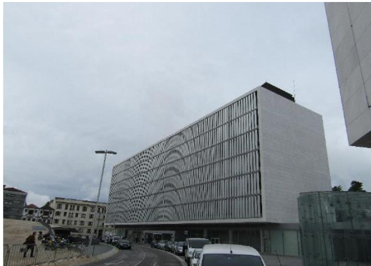
Figure 12: Porto A's office building
