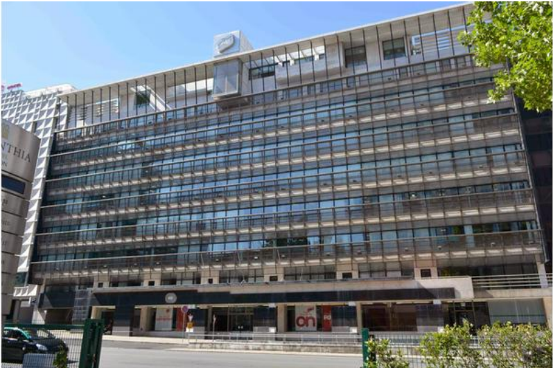
Figure 24: Lisbon Building B’s office building
